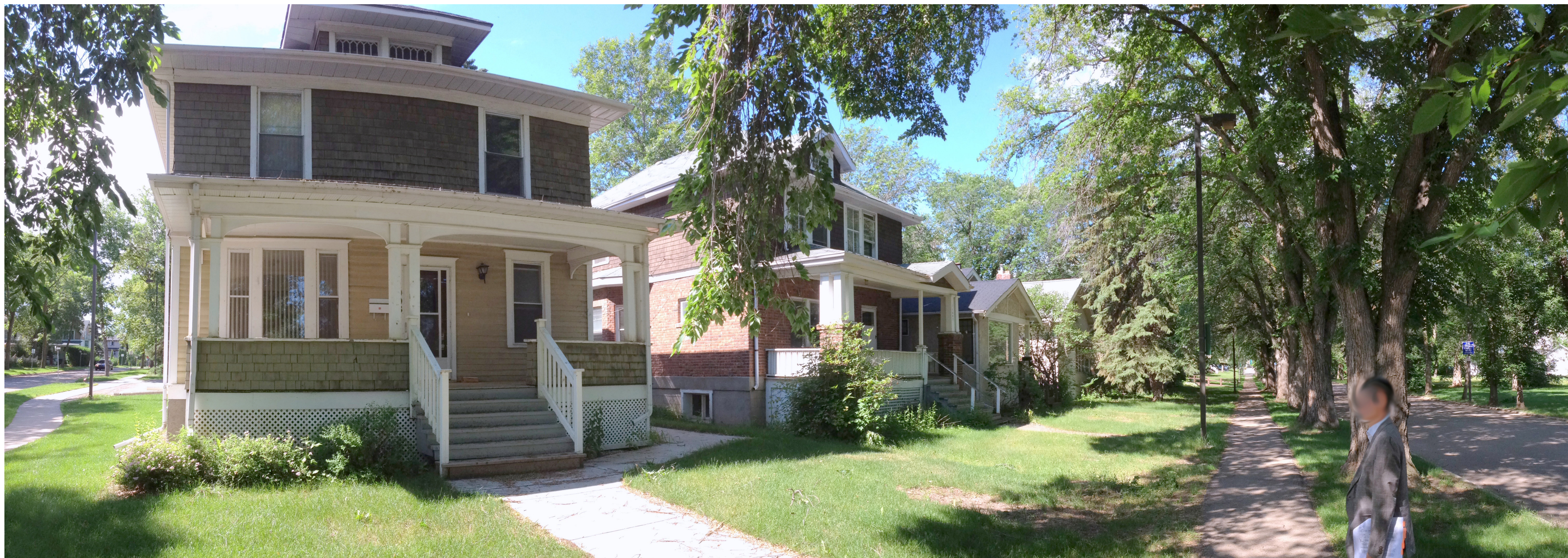
Existing houses (11003 & 11007 - 90th Avenue) retained as per preservation plan.
