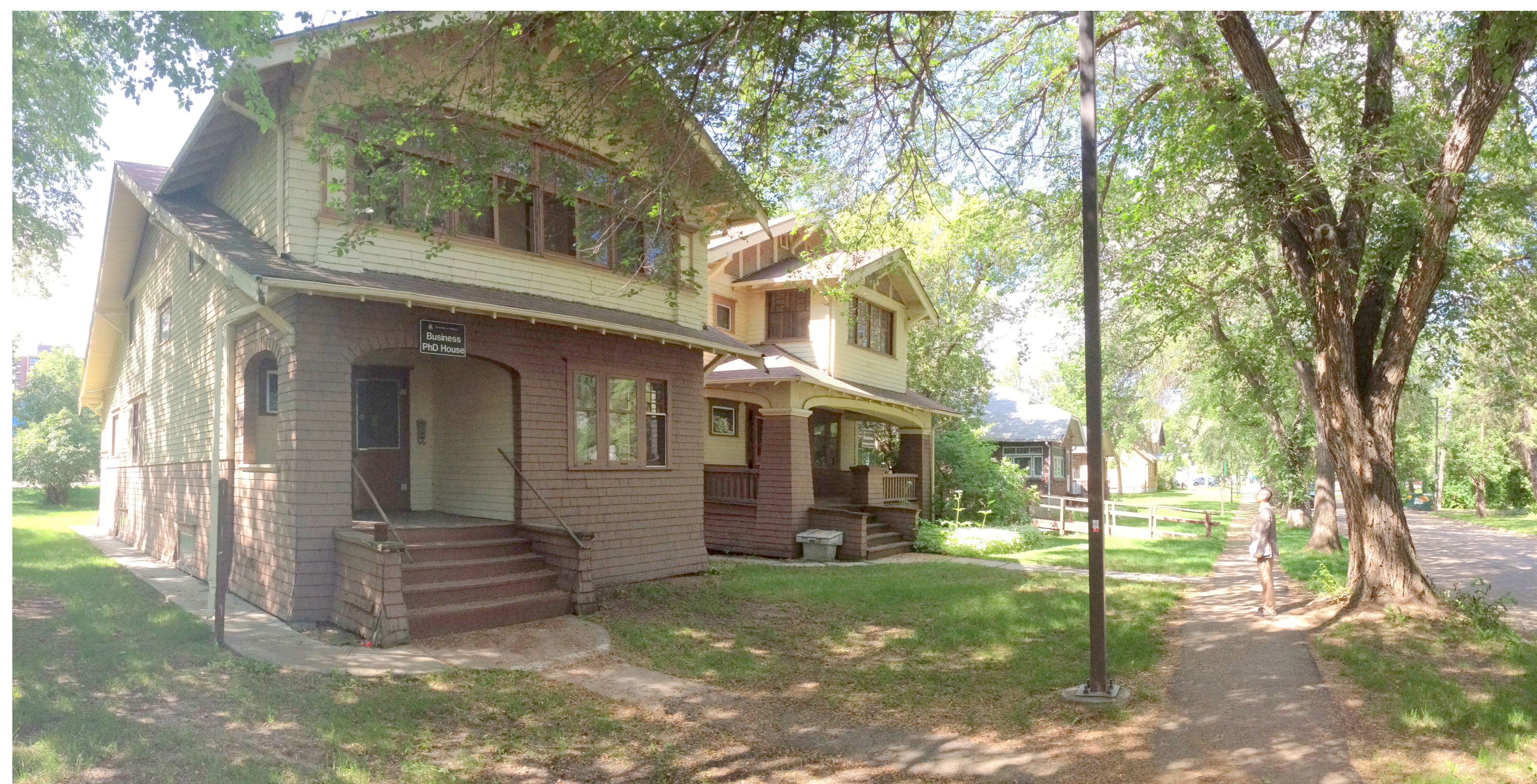
Existing houses (11019 & 11023 - 90th Avenue) retained as per preservation plan.
