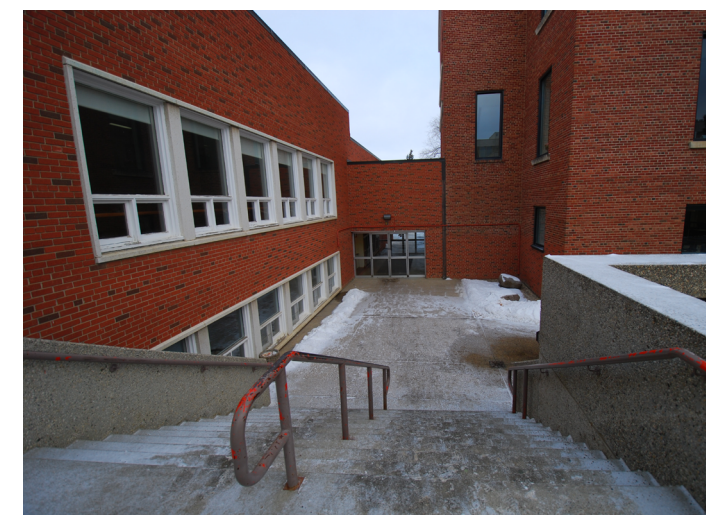
Existing University Hall Connection
