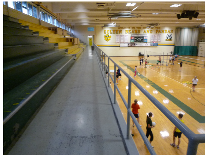
Existing Gymnasium / Viewing Area (Future Multi-Purpose Rooms / Quiet Study Space)
