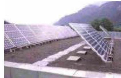
Flat Roof Installation
