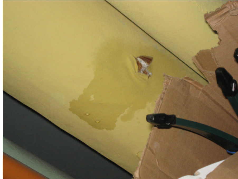
FIGURE 3: White Asbestos Containing Pipe Run Insulation
