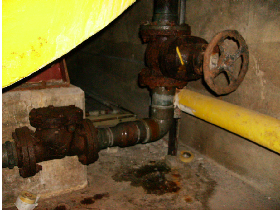
FIGURE 19: Grey Asbestos Containing Debris
