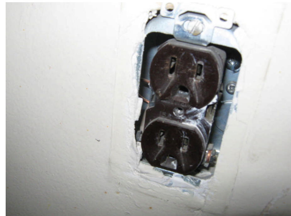
FIGURE 10: White Asbestos Containing Drywall Joint Compound
