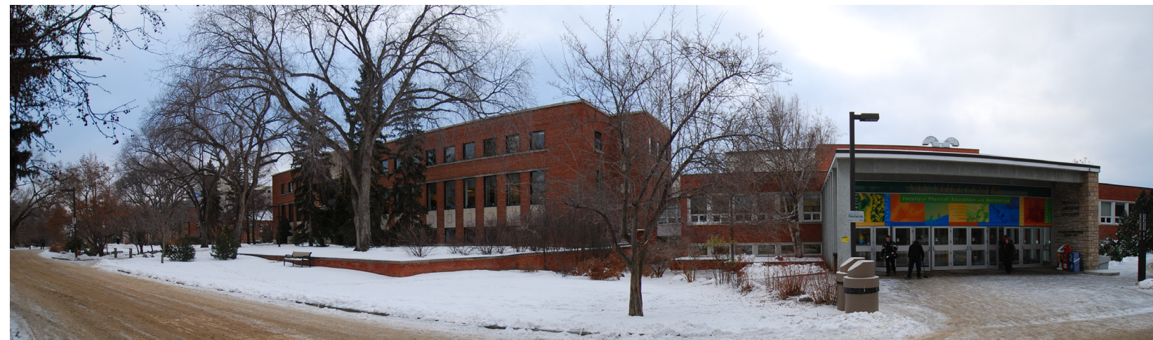
Building Exterior - North Entry
