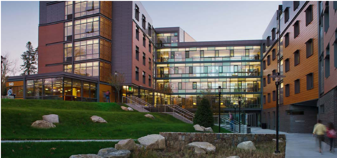
Hillside Hall at the University of Rhode Island takes advantage of a sloped site (image by LLB Architects).
