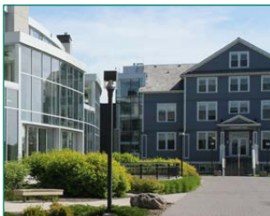
Renovation of Founders' Hall
